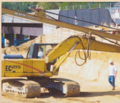
Tieback operations to secure construction walls are handled efficiently by direct drive Rineer motors turning the auger.
