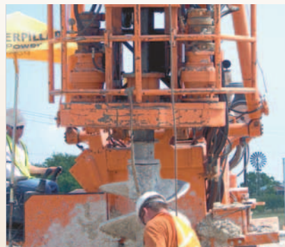
Caisson drill rigs use Rineer 4-ported motors along with a multi-speed circuit to vary bit rpm and torque.
