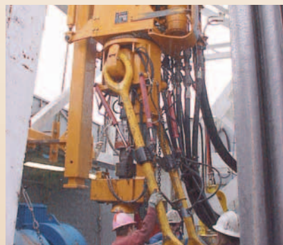
This deep well top head drive is powered by three Rineer motors plugged into the final drive ring gear.
